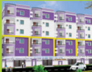
Sai Krishna Towers Penamaluru
